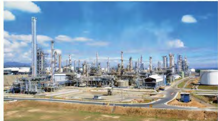
Petron Bataan Refinery
