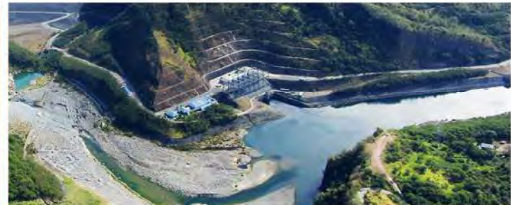
San Roque Power Plant
